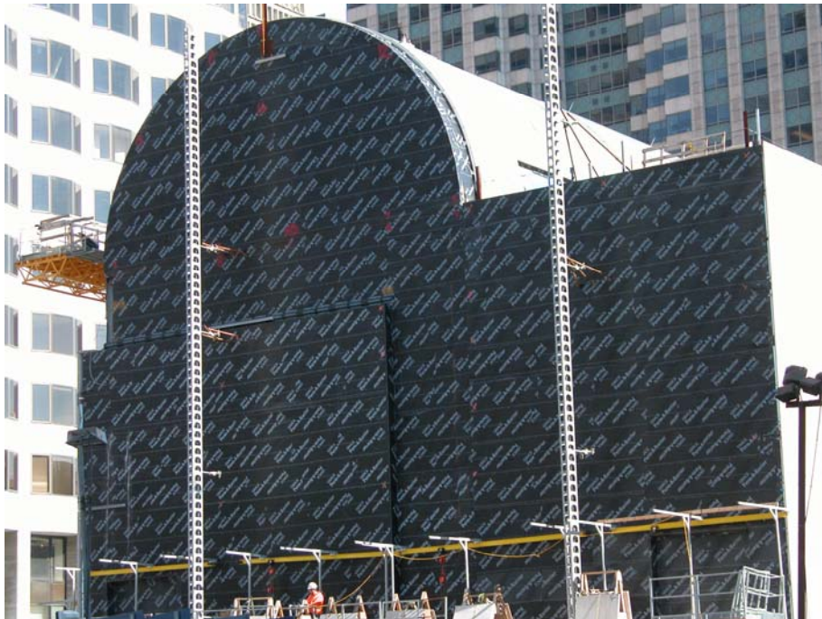
Photograph 1 – Exterior Air Barrier Using Adhered Membrane
