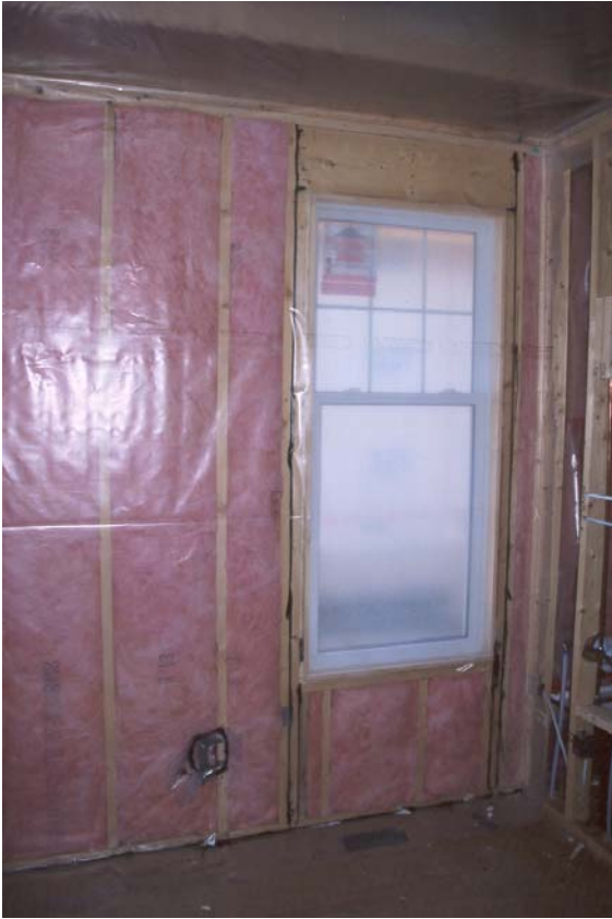
Photograph 5 – Interior Air Barrier Using Polyethylene Sheet
