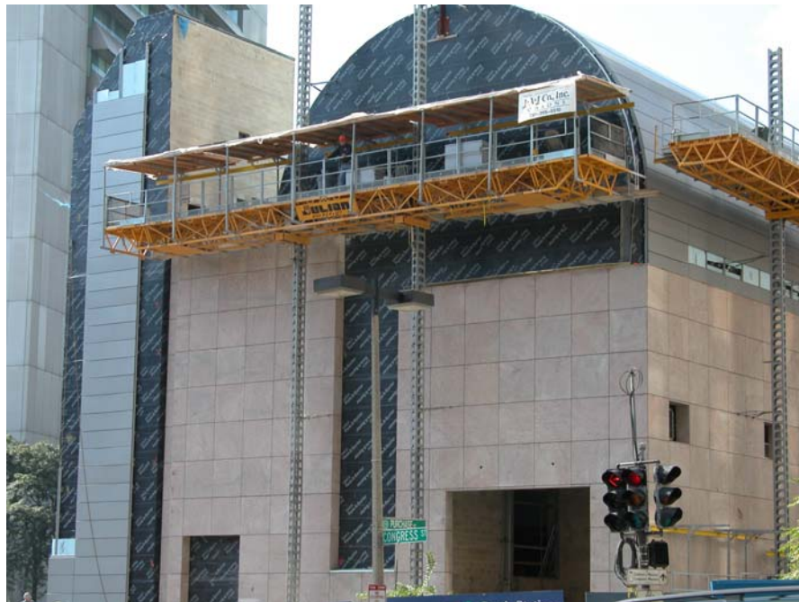
Photograph 2 – Exterior Air Barrier Using Adhered Membrane
